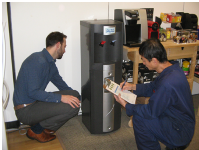
George recorded that the power supply and water valves to water coolers were turned off.
